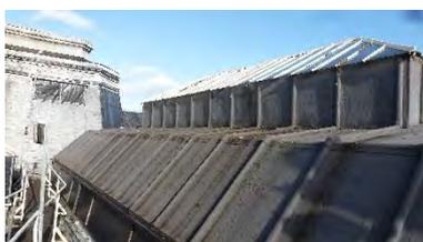
4.2.5 Roof 04b . Central . Glazed pitched and hipped lantern on vertical framework over G12 Staircase
